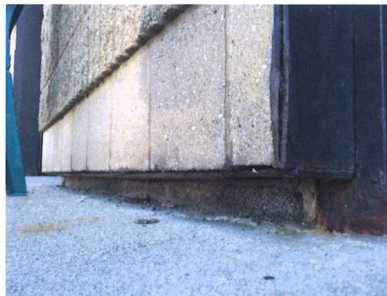
Figure 3 - Steel angle attached to block wall
