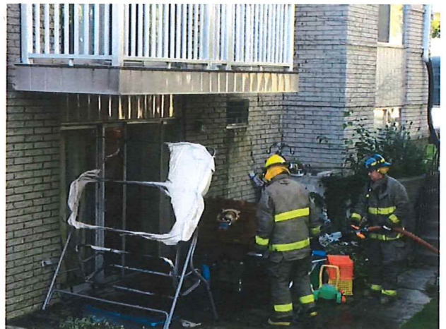
Fire outside of Kingslane Apartments on October 20 th .
