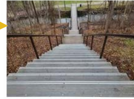
Current Condition of Stairs
