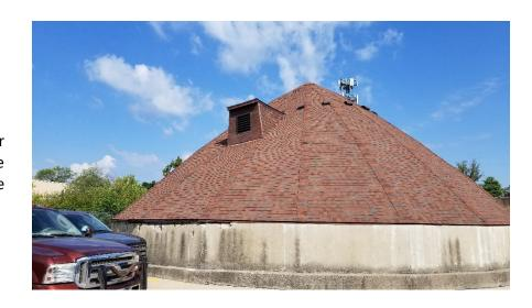
Renovation of Firearms Range - The Firearms range was built in the 1960's and is need of maintenance. The ventilation system is outdated, the automatic track that moves and faces the targets in no longer functional, and the backstop is worn to the point that ricochets are possible. To safeguard against ricochets, a mat system is used which requires regular replacement.
