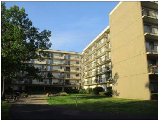
19. Back building elevation (east and north) facing south.
