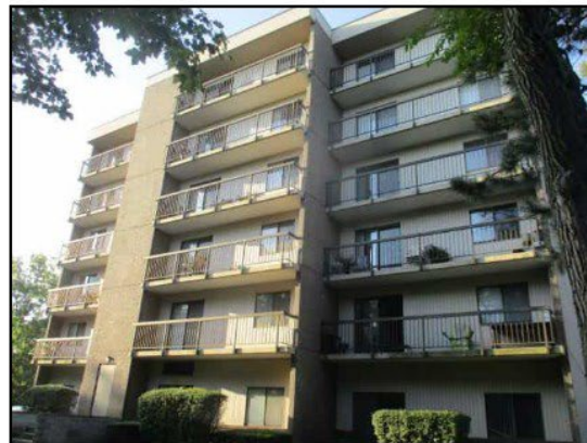
18. Back building elevation (north) facing southeast.
