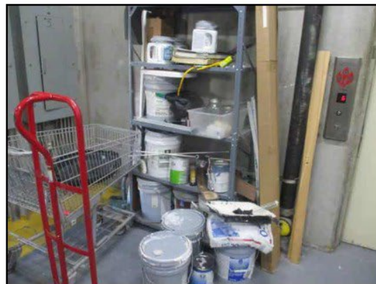
30. Paint storage in the maintenance room.
