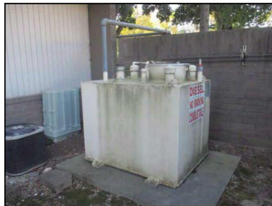
12. Two-hundred fifty (250)-gallon diesel aboveground storage tank (AST) slightly west of the southwestern corner of the Property building.
