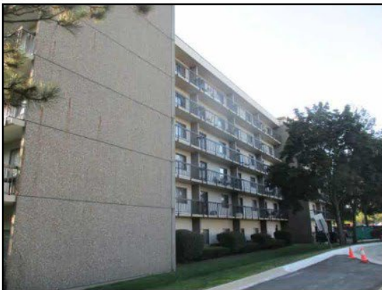
17. Side building elevation (west) facing southeast.
