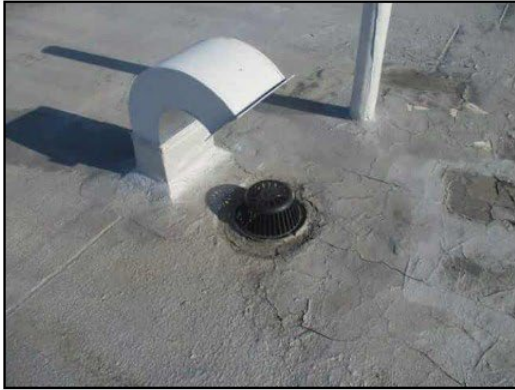
49. Typical roof drain
