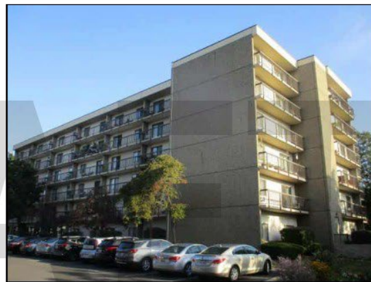
16. Front building elevation (south and east) elevation facing northwest.
