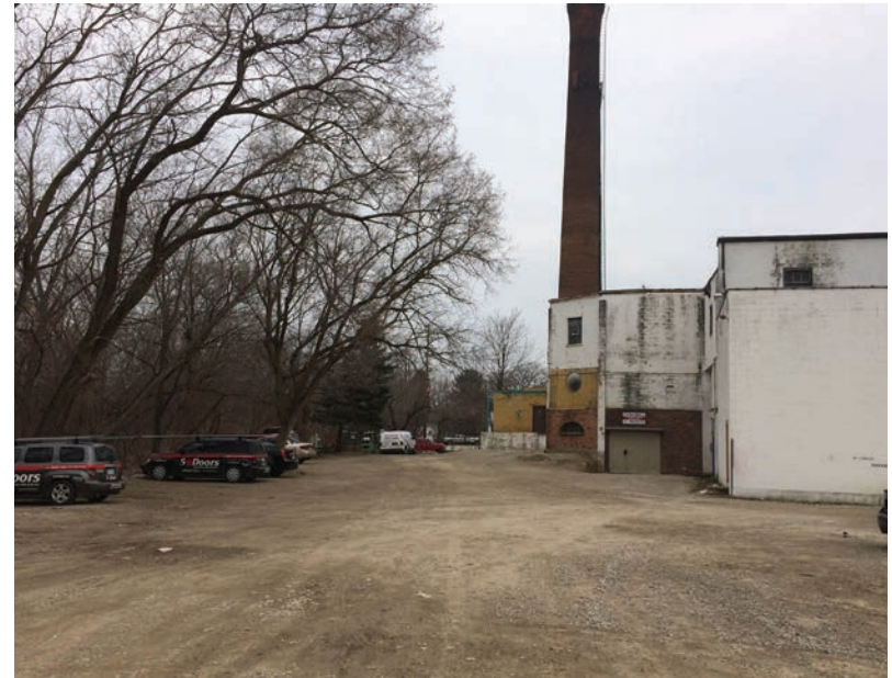
Existing lot behind the Historic Winery building
