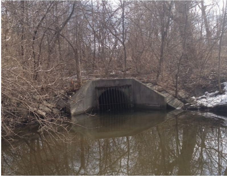
Stream channelization under 9 Mile Road
