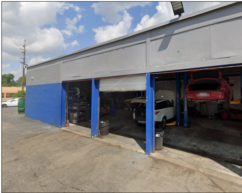
Existing conditions (Photos provided by the applicant)
