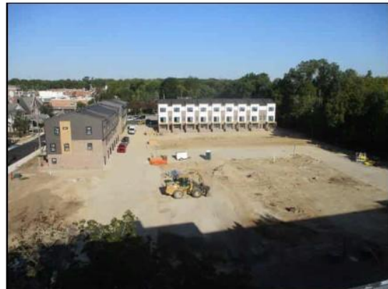
66. West adjoining residential property under construction (33000 Thomas Street)
