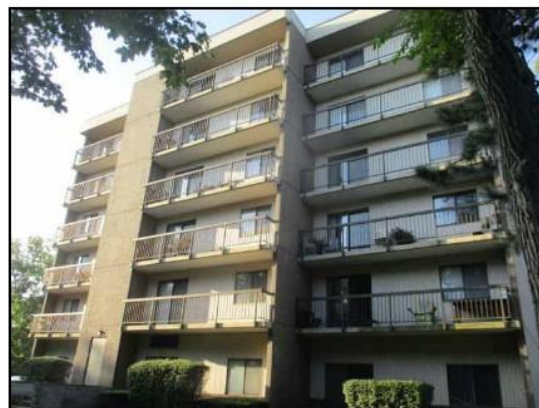
18. Back building elevation (north) facing southeast.
