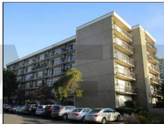
16. Front building elevation (south and east) elevation facing northwest.
