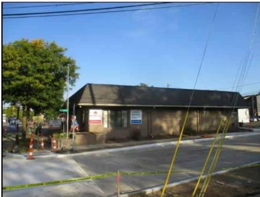
65. West adjoining office building (33004 Grand River Avenue)
