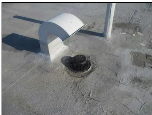
49. Typical roof drain
