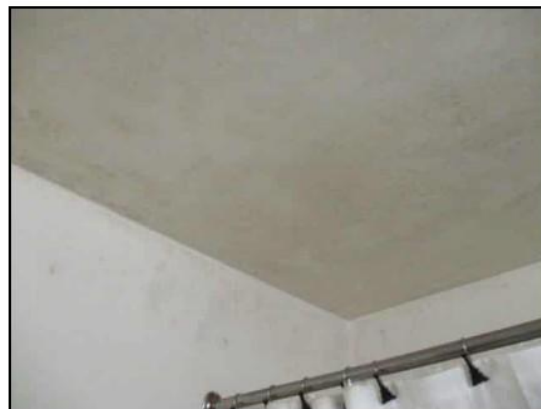
60. Suspect microbial growth in the Unit 110 bathroom
