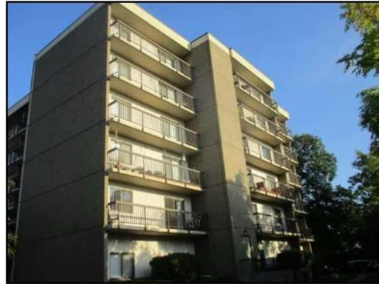
20. Side building elevation (east) facing northwest.
