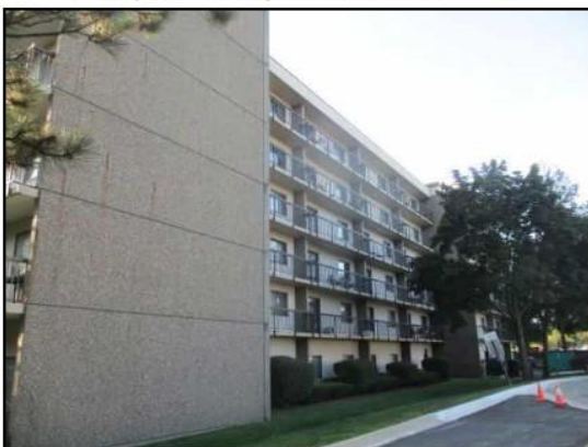
17. Side building elevation (west) facing southeast.
