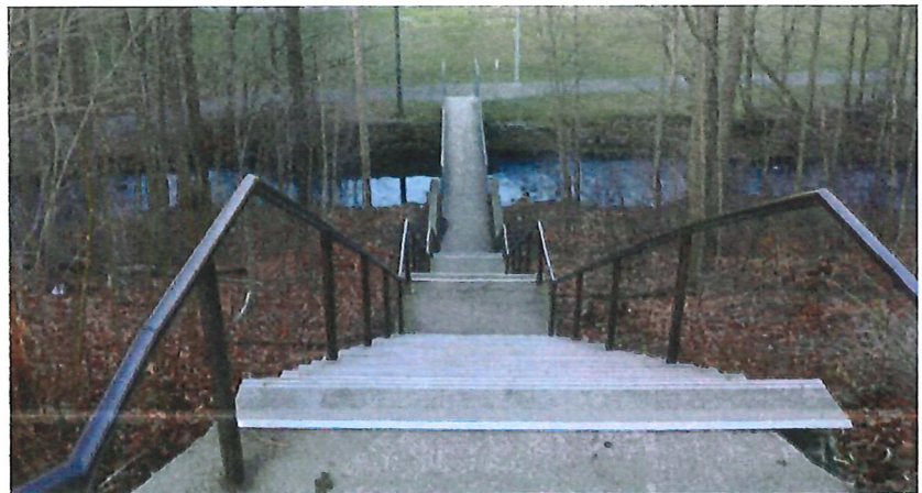
Existing Stairs to Shiawasse Park
